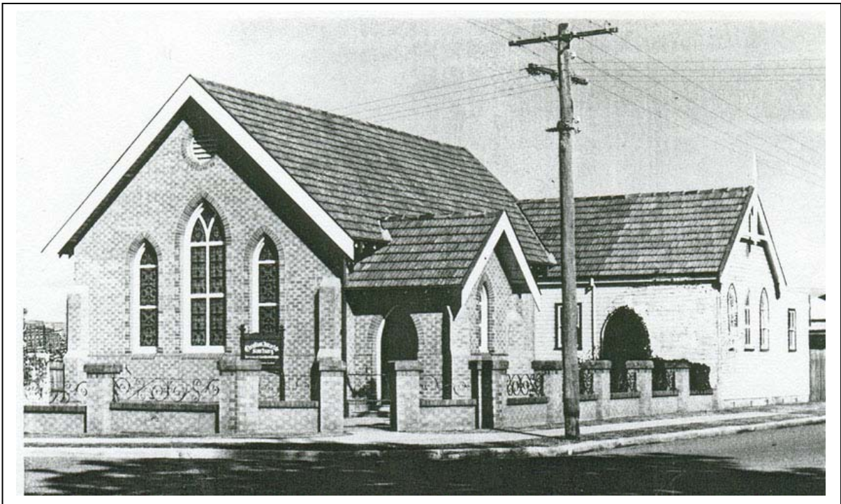
Above shows the hall at the street level and a doorway for its entrance inside the fenced area. A skillion roof had been added to the back area
