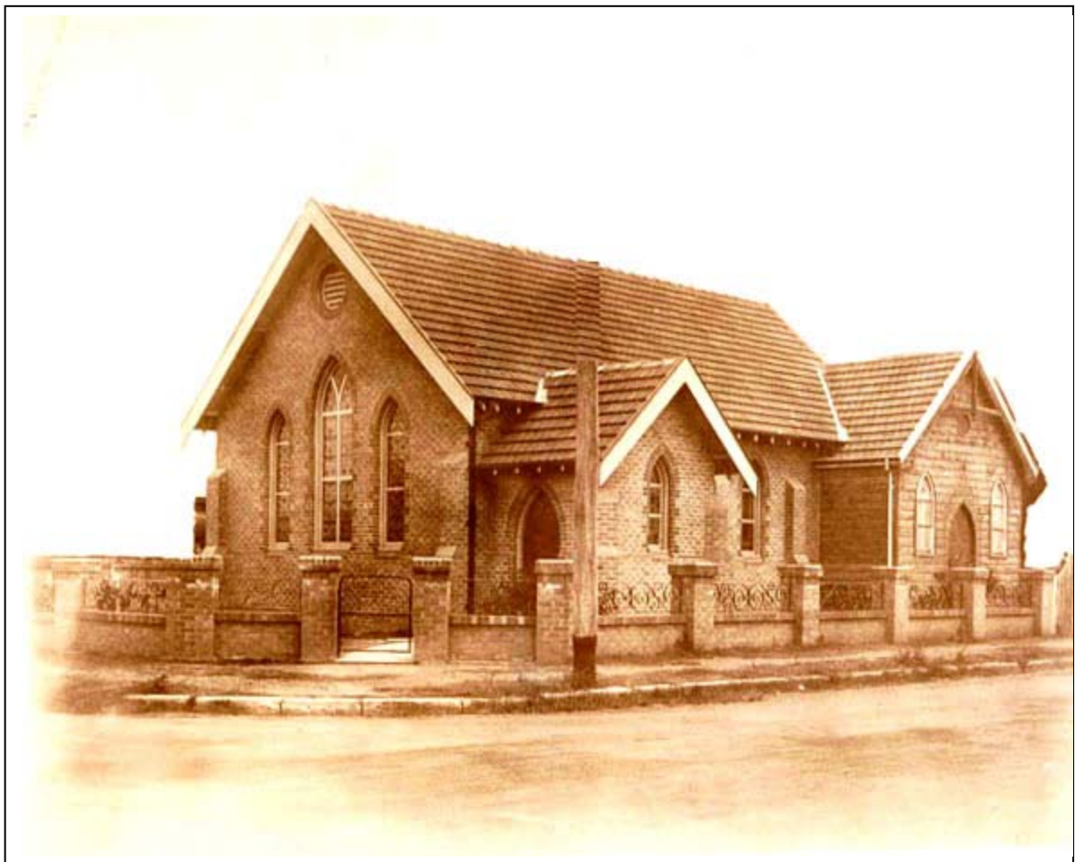
This is a picture of the finished third church.
