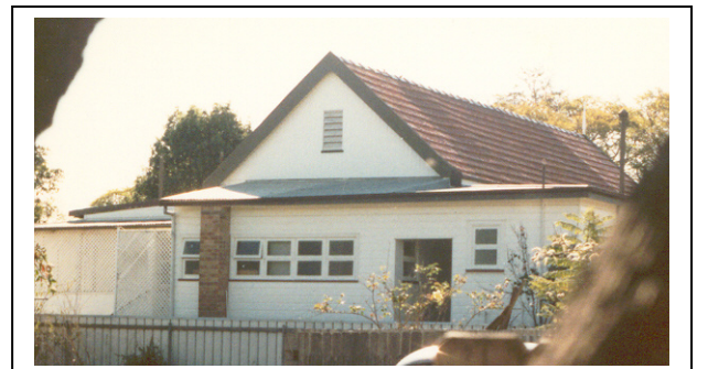
Southern side of the hall.
